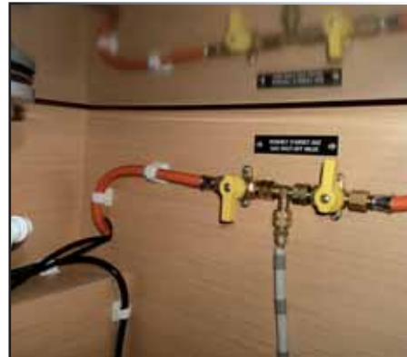
3 - HOBS AND OVEN GAS VALVES
