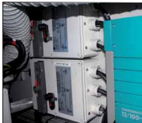
MANUAL SUPPLY SELECTOR SWITCHES COMFORT AND HIGH LOAD
