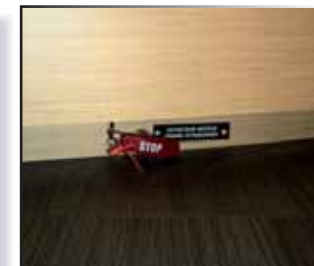
RELEASE PULL HANDLE OF 3 - PORT EXTINGUISHER 4 - STB EXTINGUISHER
