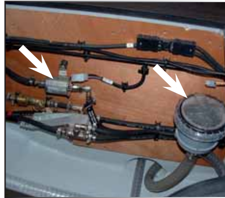
1 - FUEL BOOSTER PUMP + SEA WATER FILTER
