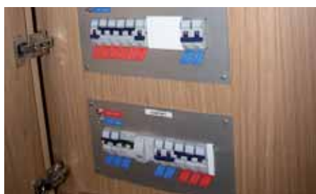
Automatic breakers 110 V - 220 V
