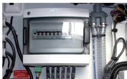
Air conditioning unit automatic breakers
